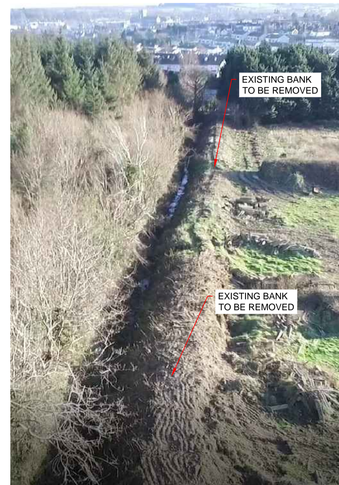
PHOTO 1 - EXISTING DRAINAGE CHANNEL
